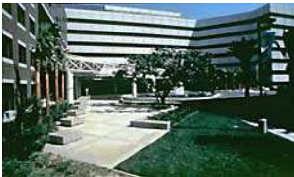
Figura 4. USC Teaching Hospital (USA). Foto: P.W. Clark
