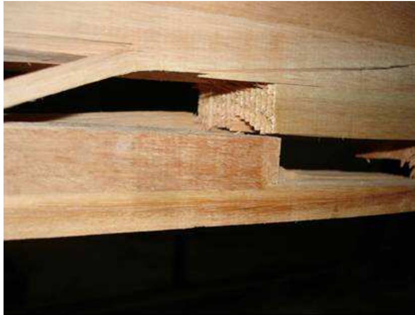
Figura 17: Finger - joints
