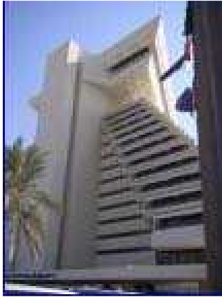
Figura 7: Hotel Sheraton, Doha, Qatar
