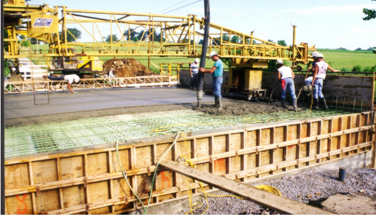
Fig. 1: Concrete placement on the Roger's Creek bridge deck
