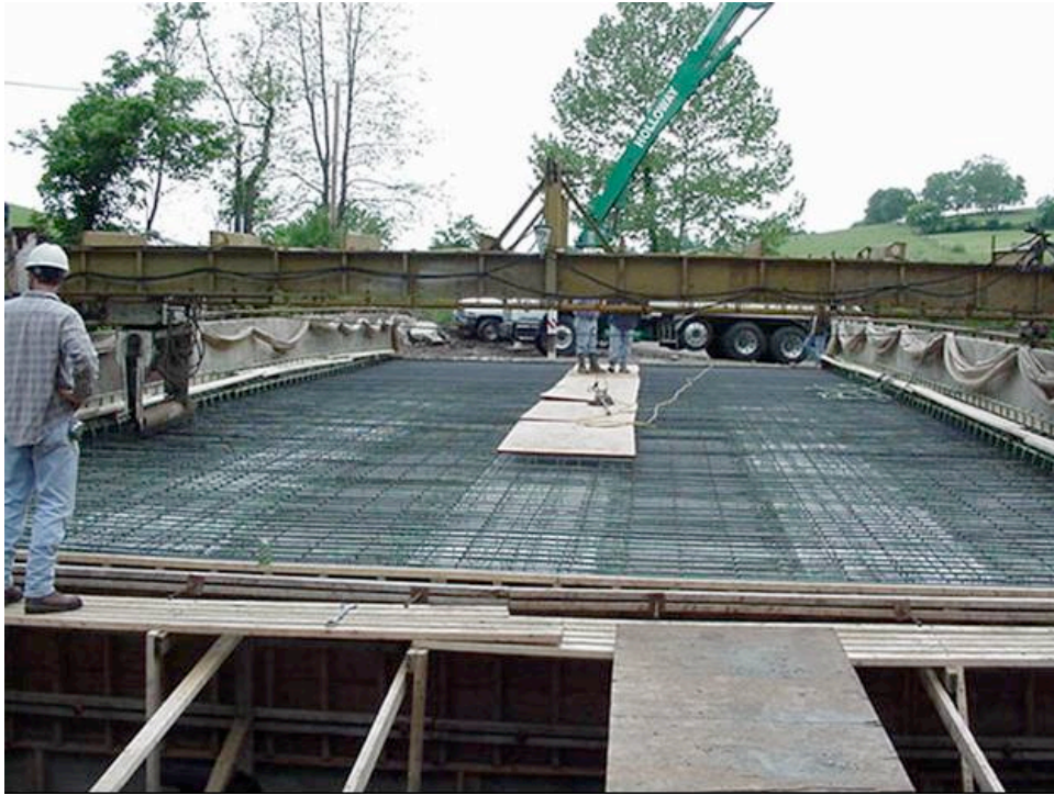
Fig. 4: The Two Mile Creek bridge deck prior to concrete placement
