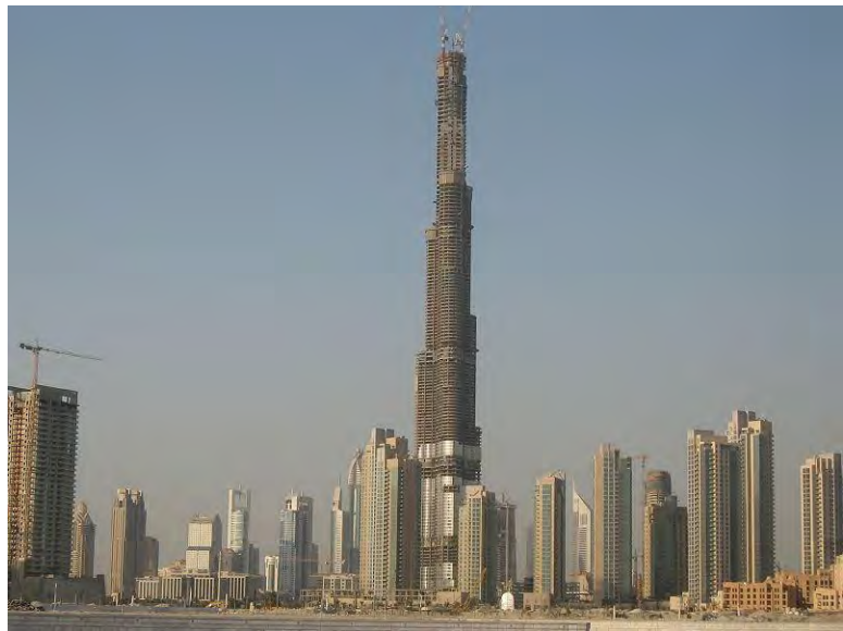
Figure 13: The huge Burj Dubai residential tower in UAE is likely to be instrumented for windspeed and building motion when completed.
